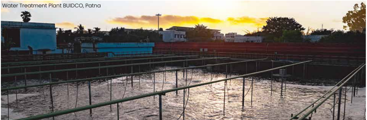
Water Treatment Plant BUIDCO, Patna
