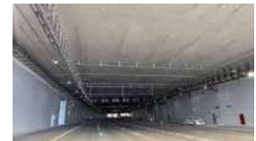
Mina Zayed Tunnel - Abu Dhabi
