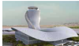
Fujairah International Airport Expansion
