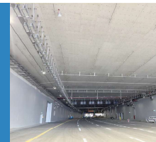
Mina Zayed Tunnel – Abu Dhabi
