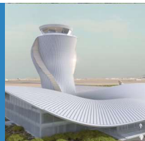
Fujairah International Airport Expansion
